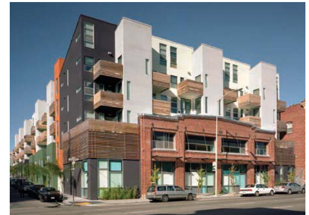
The façade of this historic structure is preserved while allowing for new housing behind.
