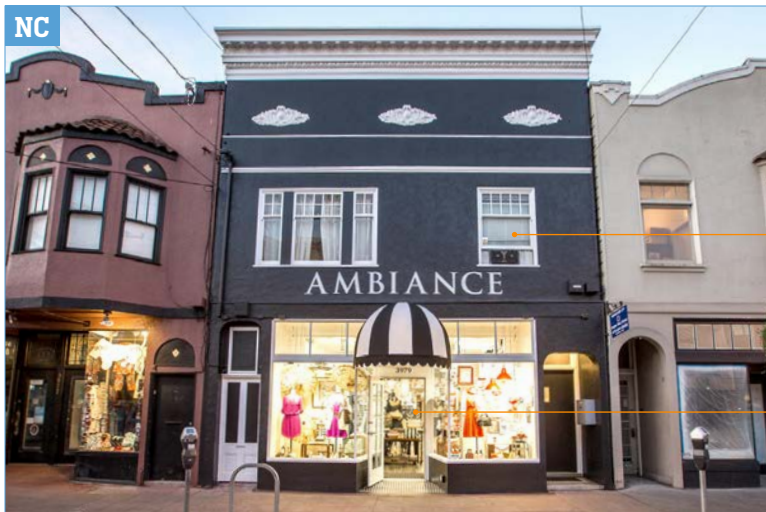
Neighborhood commercial streetwalls should be present at the sidewalk.
