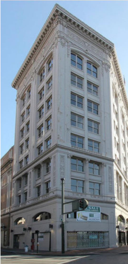
Detail and depth on the top story can help terminate the building.
