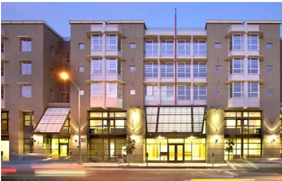
Coordinated lighting, signage, sunshading, storefronts, and canopies enliven buildings.
