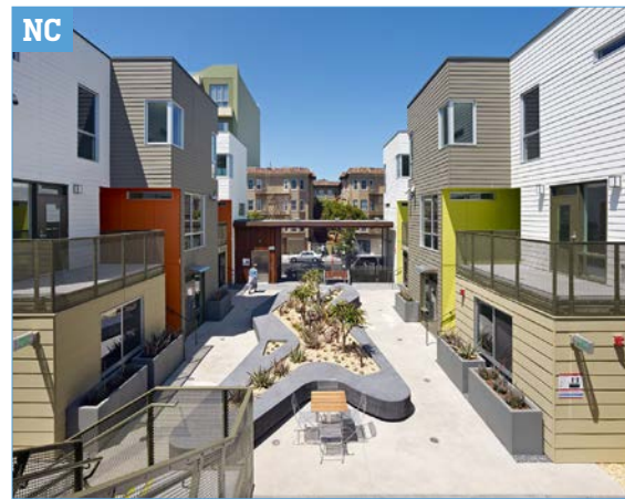
Sculpt and detail building mass to add richness and spatial variety to frame open space.
