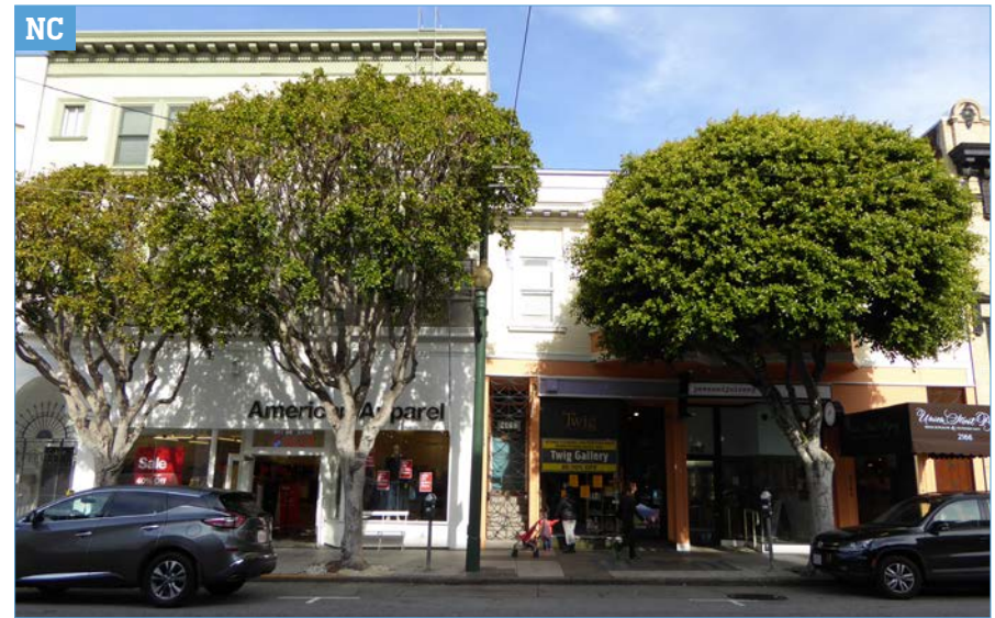
Street trees help shade buildings and reduce solar heat gain.
