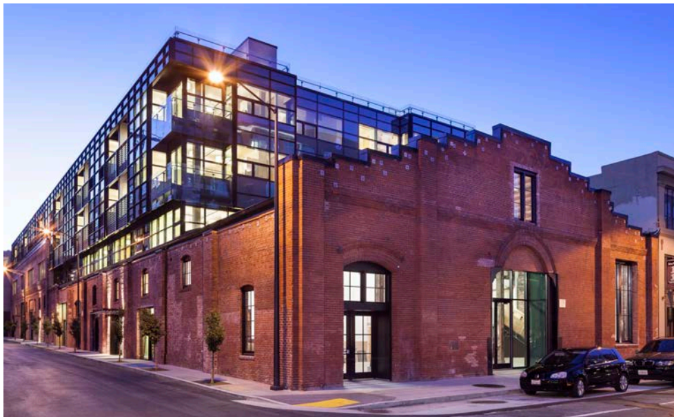
Concepts can structure the relationship between new and historic structures and highlight their best features.
