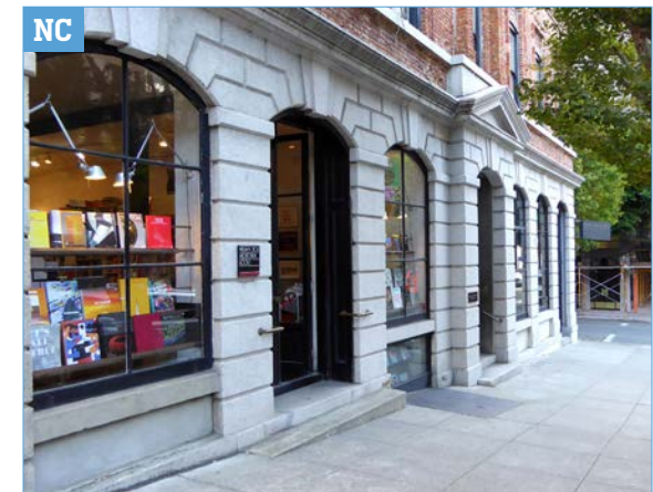
Add smaller, human-scaled features at the ground where they can be easily seen.
