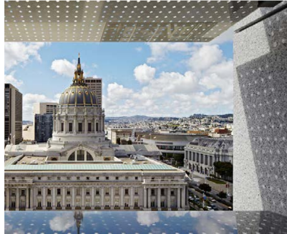
Light shelves help protect interiors from heat gain while bringing daylight into interior space.
