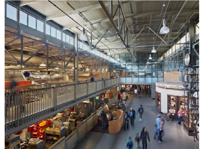
Reuse existing buildings and clerestory daylighting to reduce resource and energy use.
